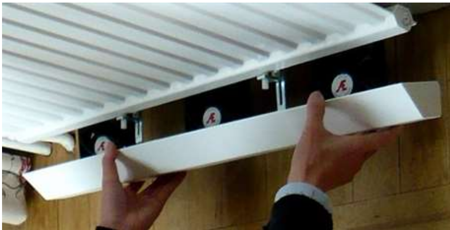
Figure 1. Add-on-fan placed on a single-panel radiator (elementflakten.se, 2016)
